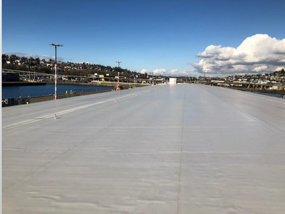
T-91 Building C-173 Roof Overlay
